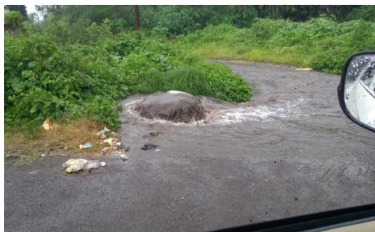
Fig 2. Overflowing of the manhole during rainfall.
